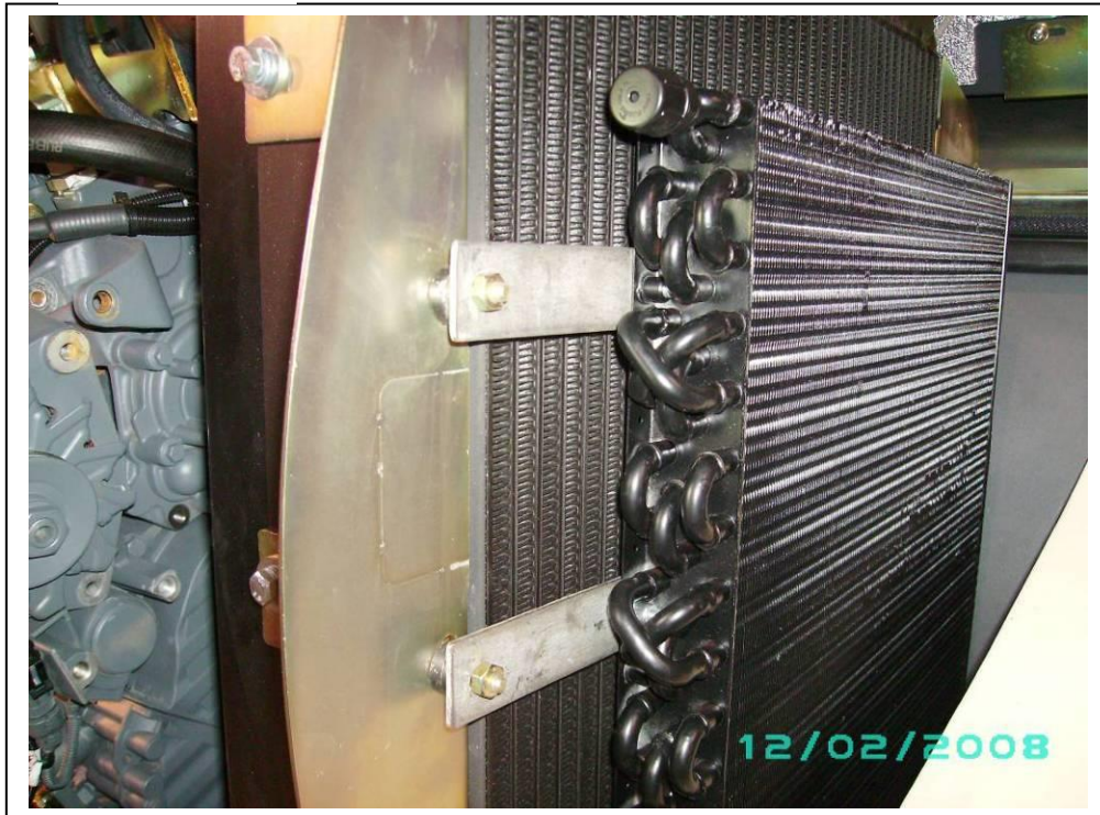
Fitting side of the condenser showing brackets bolted in place. Brackets are shipped loose.
